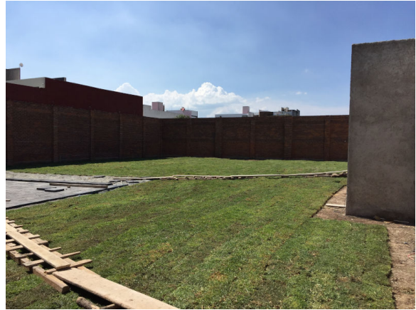
The sod has been planted for the garden.
